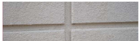
Photograph 8: Finished panel cladding joint.
