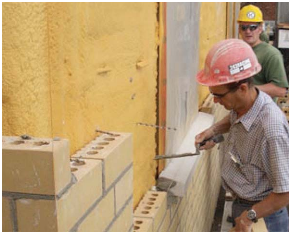
Photograph 3: Brick Installed—Step two.
