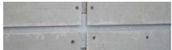
Photograph 7: Panel Cladding Joint Treatment—Joints do not need to be watertight or airtight as cladding system is back-ventilated and drained.
