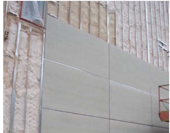
Photograph 5: Vertical channels for panel cladding.
