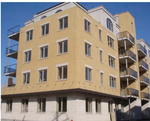
Photograph 4: Finished Building—Step three.
