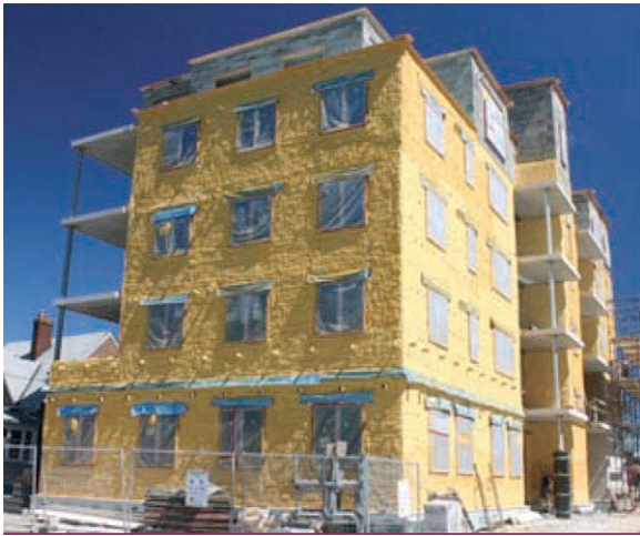
Photograph 2: SPF Applied—Step one.
