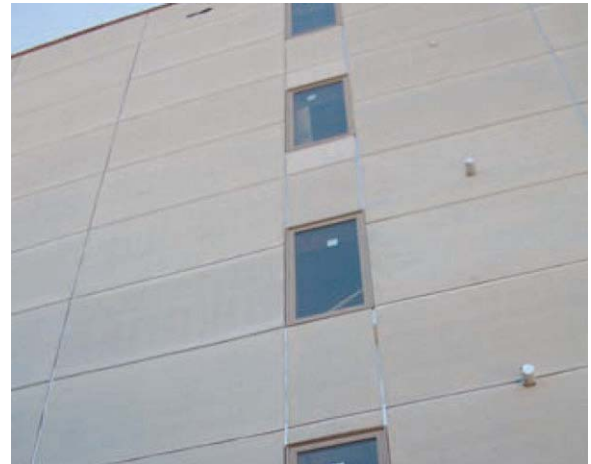
Photograph 6: Panel Cladding—Fiber cement panels attached to metal channels.
