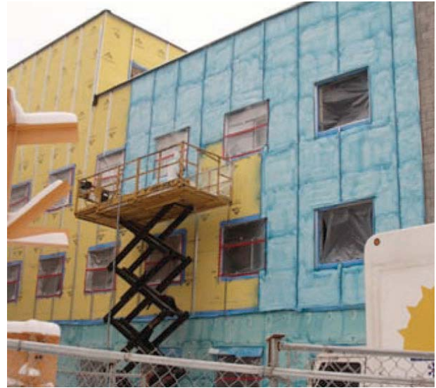
Photograph 9: Z-Bar attachment for panel cladding.
