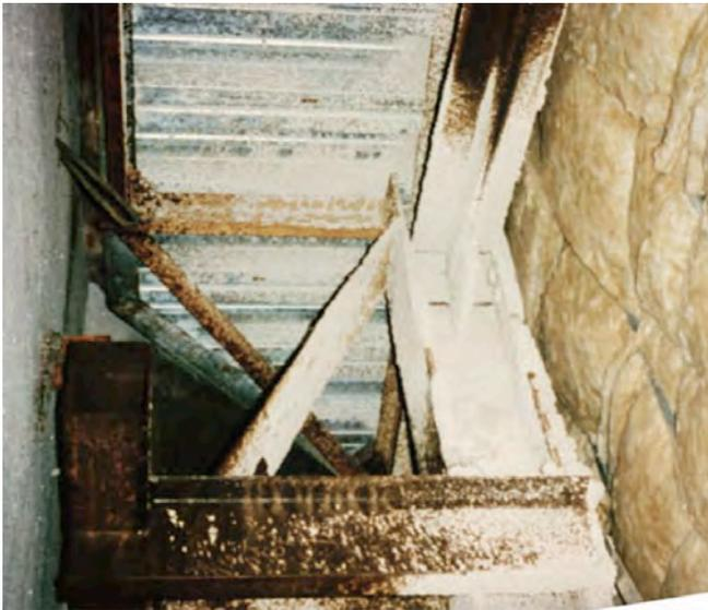
**Photograph 5: Gift from the Engineering Gods—A continuous perimeter air gap between the precast panels and the interior insulated steel stud wall framing.**
