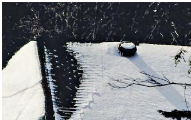
**Photograph 7:** Attic supply fan pressurizing roof cavity.
