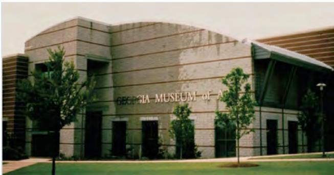
**Photograph 8:** Fire hose wetted reservoir cladding.
