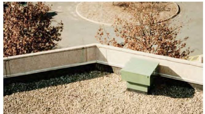
**Photograph 6: Rooftop interstitial cavity pressurization system.**
