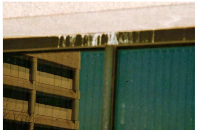
**Photograph 3:** Condensed water leaking out at window heads.
