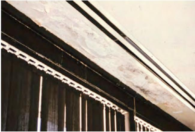
**Photograph 4:** Water damaged interior finishes at exterior walls.
