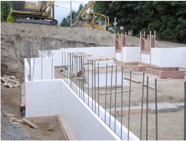
Photograph 3: Foam Building Blocks —Stack 'em up and fill 'em with concrete.
