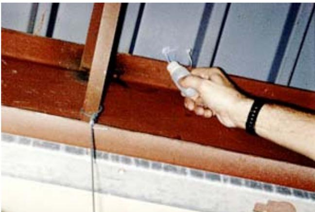
**Photograph 9:** Sucking on a Wall Part Deux—Commercial return plenum draws air out of exterior walls into the return side of the HVAC system and then subsequently connects to the breathing zone of the occupied space.
