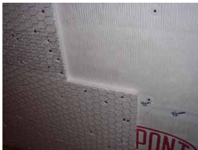
Photograph 9: Water-Managed Claddings —Note the “crinkled” housewrap providing relief of hydrostatic pressure, providing lateral “hygric redistribution” and protection of the OSB (i.e. the de facto “water control layer”). Stucco can be applied directly to the foam, or any other cladding.
