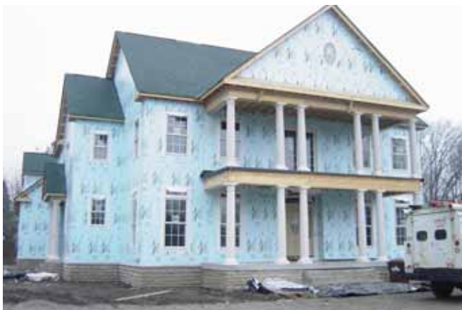
Photograph 2: Upstart? —Fifty years as a sheathing but still considered an upstart. Extruded polystyrene (XPS) completely sheathing the structure – continuous thermal break. “Beginning show up on the range...confusing the cowboy builder and architect...”
