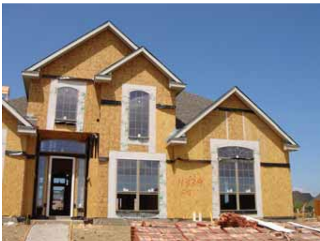
Photograph 1: Ubiquitous Sheathing —A pretty familiar sight – a home completely sheathed with oriented strand board (OSB); “ruling the range...”
