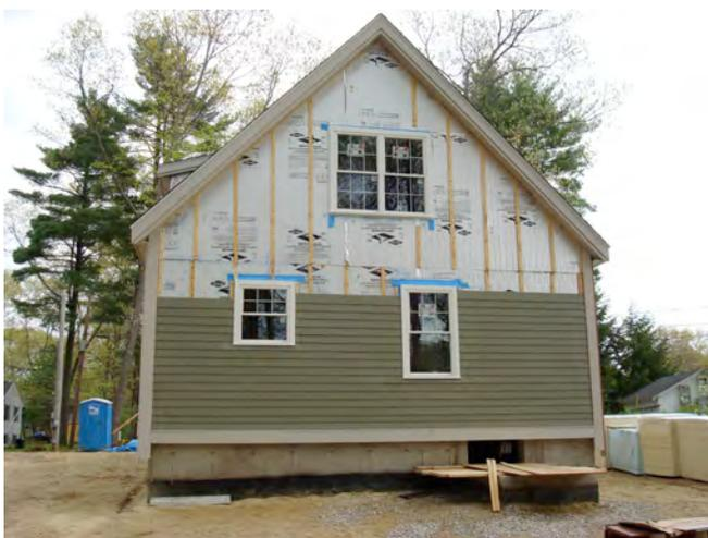
**Photograph 7: Furring**—When foam sheathings exceed 2 inches in thickness 1x4 furring becomes necessary. This wall has 4 inches of foil-faced polyisocyanurate insulating sheathing installed over a 2x6 wood frame wall. The wood furring acts as the nail base for the fiber-cement cladding.
