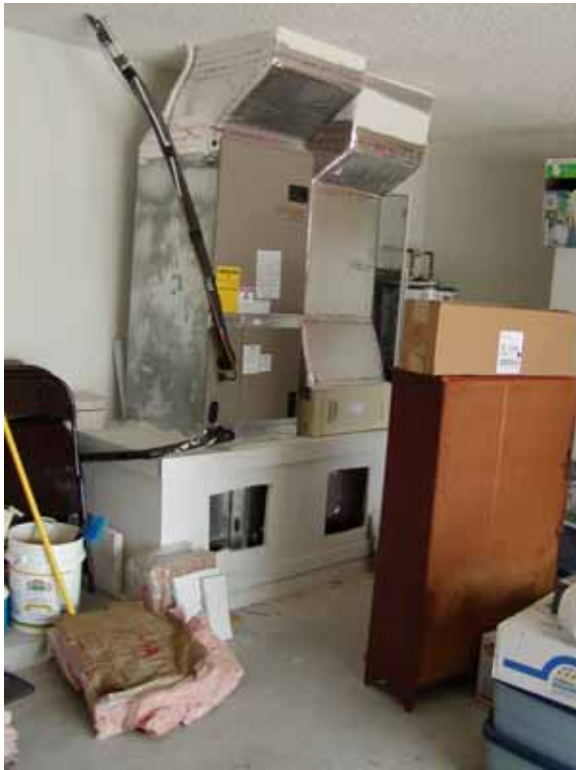
Photograph 6: Garage Return Platform —After a vented attic what is the worst possible place to locate an air-handler? Yes, you guessed it, the garage. Florida HVAC at its best.
