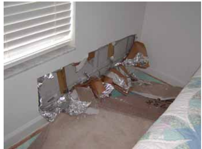
Photograph 1: Unique Florida Experience —Baseboard gets moldy, gypsum board at baseboard gets moldy, kraft paper facing of reflective foil gets moldy...
