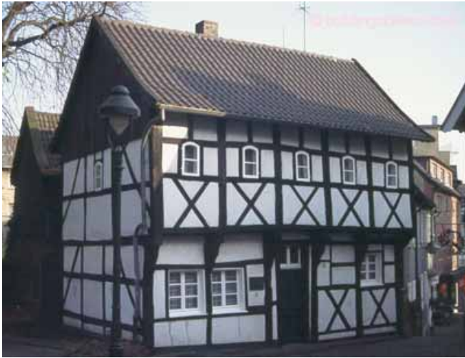
Photograph 4: Waltrop House —Germany, 1400, wattle-and-daub infill panels with an exposed timber frame. Wattle-and-daub has a lime plaster coating. Timbers are coated with tar.
