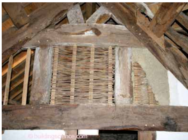
Photograph 3: Wattle-and-Daub —This is a timber frame house in Wales, United Kingdom, with the wattle-and-daub exposed. Note the weaving of the wattle.
