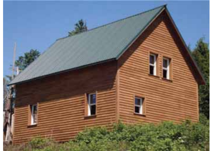
Photograph 1: Extreme Enclosure —“Superinsulated” does not do justice to this house constructed by the Hydaburg Tribe in Alaska that is ultra-airtight and ultra-vapor tight (less than 0.5 ach at 50 Pa [0.20 in. w.c.] and less than 0.5 perms).
