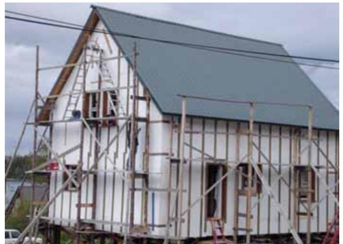
**Photograph 2: Exterior insulation**—Multiple layers of rigid insulation on the exterior of a wood-frame structure held in place with wood furring strips. Note the inset location of the windows allows the water management layer of the window to connect to the water management layer of the exterior wall (the fully adhered membrane).
