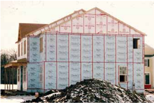
Photograph 6: Insulating Sheathing - With insulating sheathing the water control layer is the exterior face of the insulating sheathing taped.
