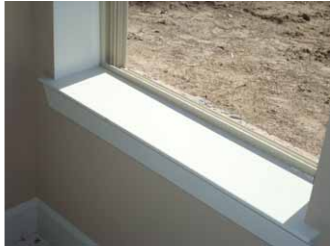
Photograph 9: Deep Window Openings - The combination of advanced framing and insulating sheathing leads to deep window openings. Window returns are typically gypsum board with wood trim only at the bottom.
