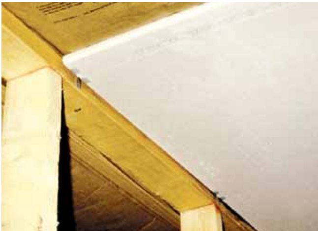
Photograph 4: Gypsum Board Support – Drywall clips result in floating corners, a good thing, as drywall cracking is reduced.
