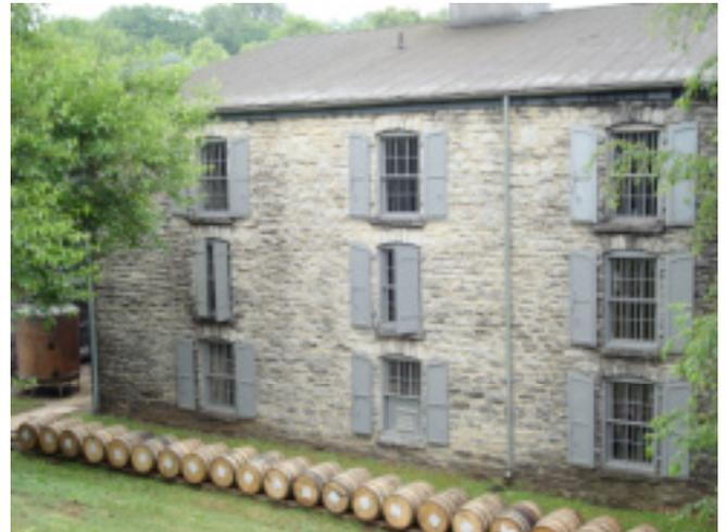
**Photograph 5: High Mass Warehouse**—Metal roof over timber deck, stone walls, dirt crawlspace, cross ventilation and stack ventilation. The temperature of the ground and the thermal resistance and thermal mass of the walls moderate the temperature swings within the building. The metal roof is cooler than asphalt shingles or a built up roof.
