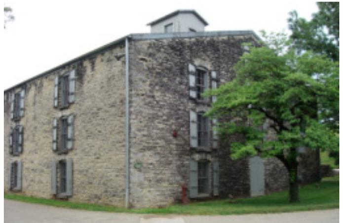
**Photograph 9: “Angels Share”**—Legend has it that the mold growth on the exterior of old bourbon warehouses is due to the evaporation of alcohol from the barrels and the subsequent diffusion of this alcohol through the walls providing nutrients to support mold growth. The “missing” alcohol from the barrels is called the “angels share”. Of course sometimes mold is just mold (yes, sometimes a cigar is just a cigar...).
