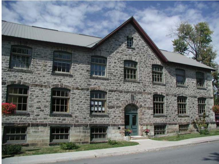
Figure 6: This old enclosure controls rain penetration by storing moisture in many layers of masonry. Note that overhang and window details shed rain off the surface, thereby reducing the amount of rainwater that needs to be stored between wetting events.
