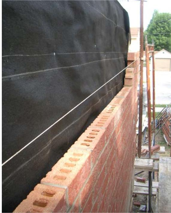
Figure 8: Drained brick veneer, employing lapped building paper as the drainage plane
