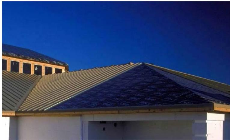
Figure 4: Metal-cladding is being placed over a concealed barrier (a waterproof fully-adhered "self-sealing" membrane) to form the rain control system of this sloped roof.
