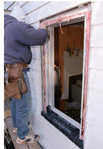
Insulation was installed around the window opening. The membrane pan flashing installed to receive the replacement windows was extended upwards and wrapped the entire opening.
