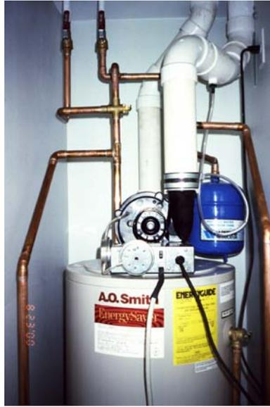
Photograph 2: Domestic Hot Water: Sealed combustion gas water heater provides domestic hot water.
