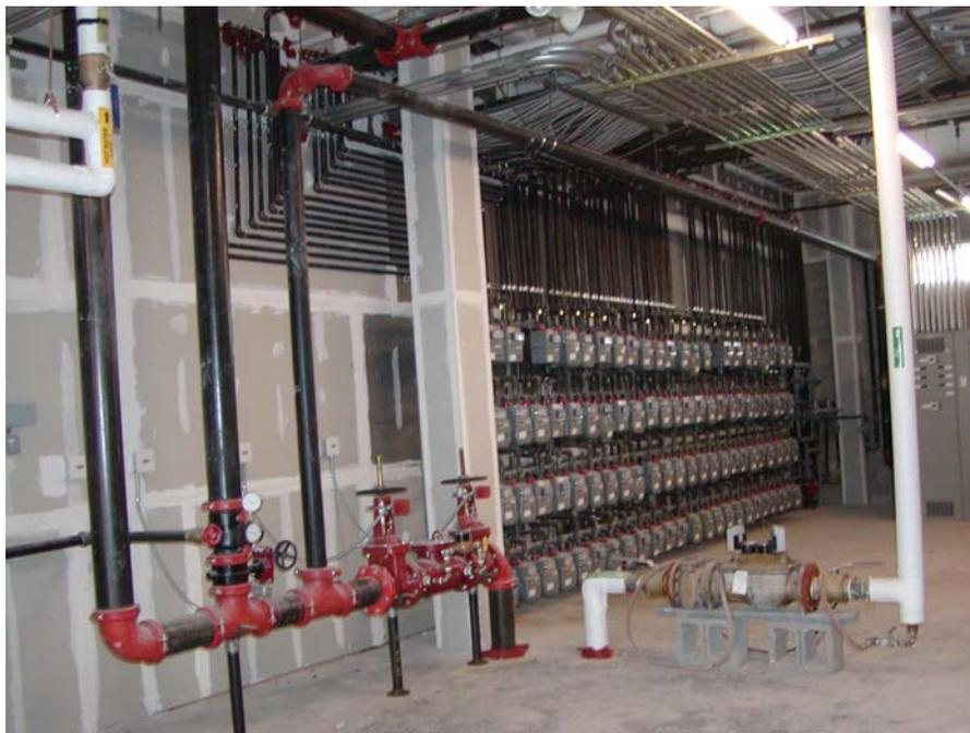
Photograph 5: Individual Gas Metering: Gas for space heating and domestic hot water is separately metered to each individual unit.
