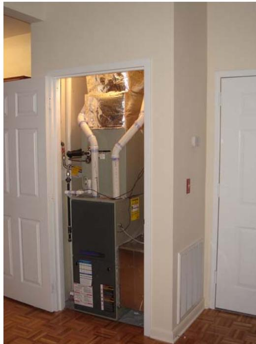
Photograph 1: Space Heating: Sealed combustion gas furnace provides space heating.
