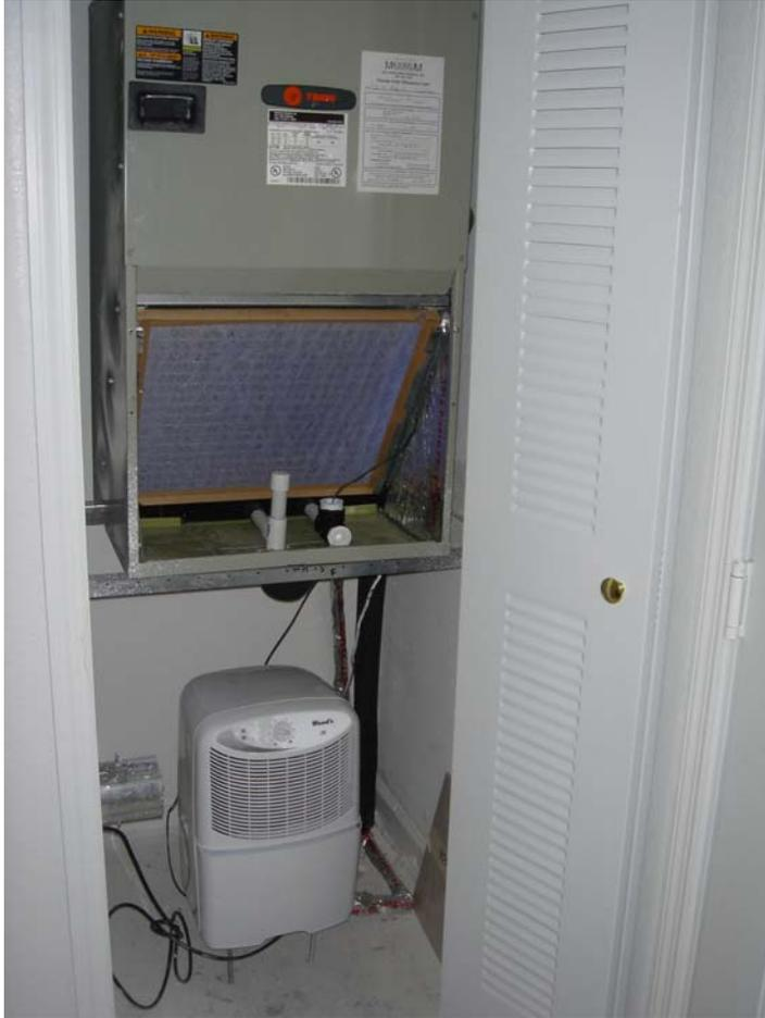
Photograph 6: Part Load Humidity Control: Individual dehumidifiers are provided in each unit – typically in the air handling closet – to handle part load humidity in hot humid climates.
