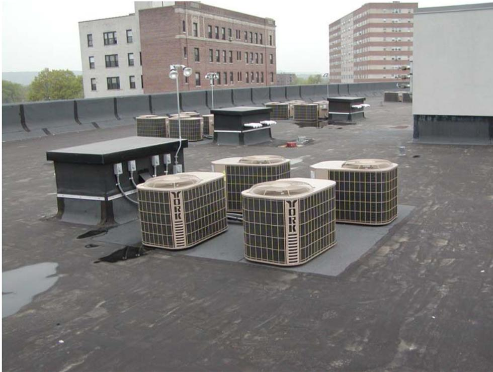
Photograph 3: Services Located on Roof: Rooftop penetrations are collected and located in “doghouses” – all cable, duct and pipes are run through walls of “doghouses”.
