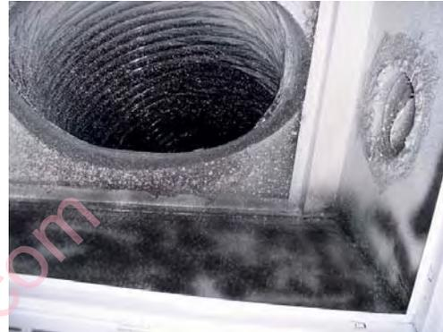
Outside air duct connected to return duct; note outside air damper on right
