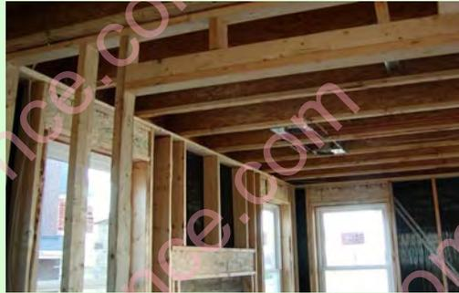
Above: Single top-plate, 24-inch o.c. in-line framing and metal cross bracing
