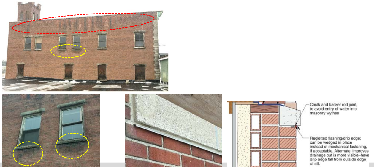
NESEA BE21: Moran Square-Low Carbon Renovation
