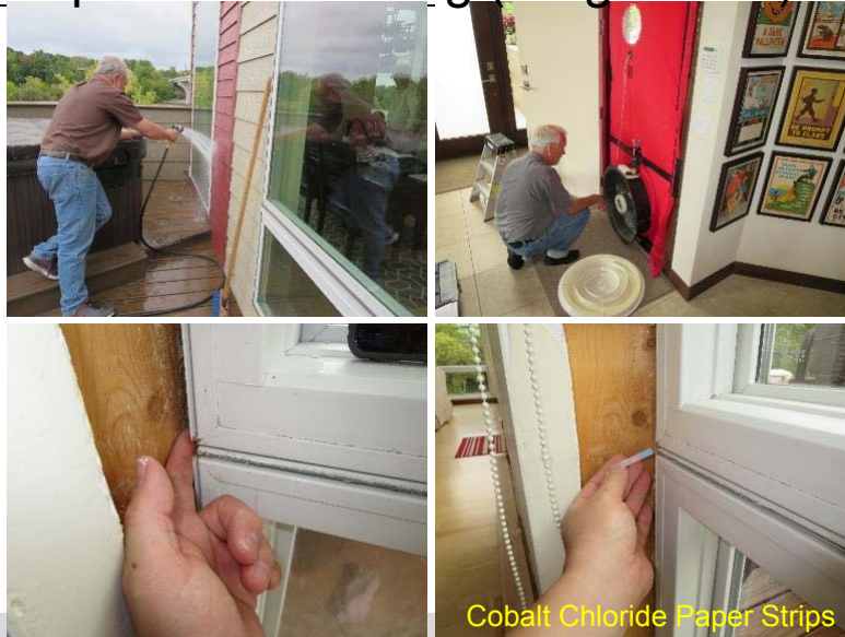
Tools of the Trade for Building Diagnostics
