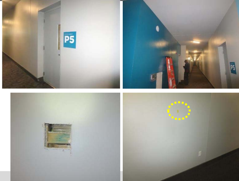
Tools of the Trade for Building Diagnostics
