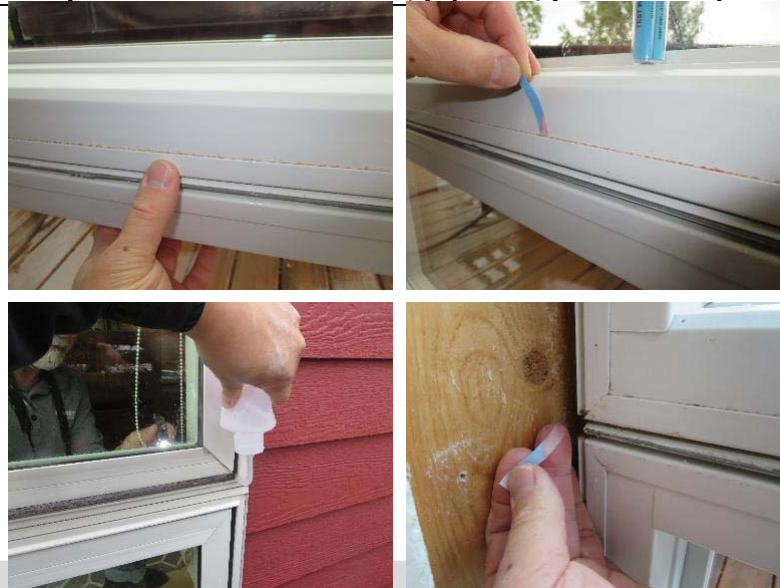
Tools of the Trade for Building Diagnostics
