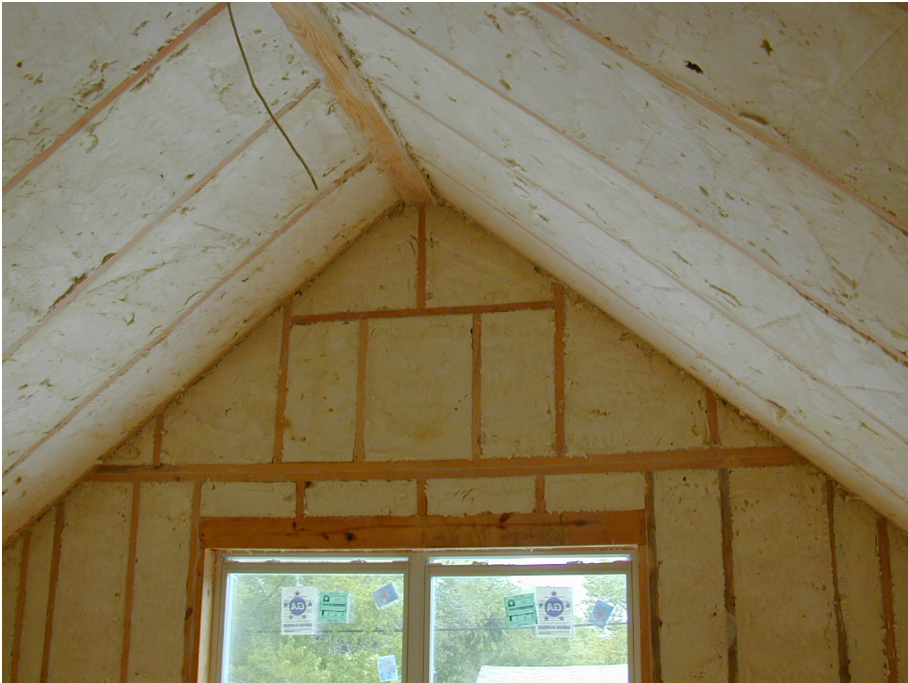
Photograph 2: Spray Foam Insulation
