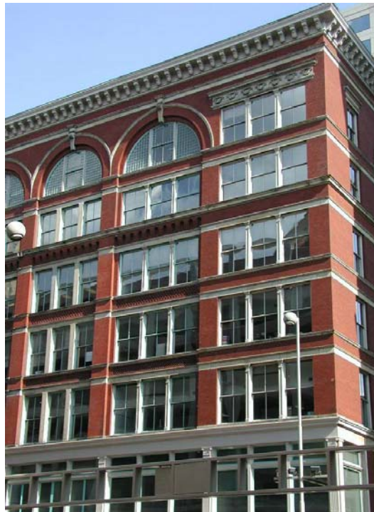
Photograph 3: Solid masonry office with generous window area, and fine detailing. Durable, strong, and functional, with moderate R-value, this type of building was common after the Industrial Revolution
