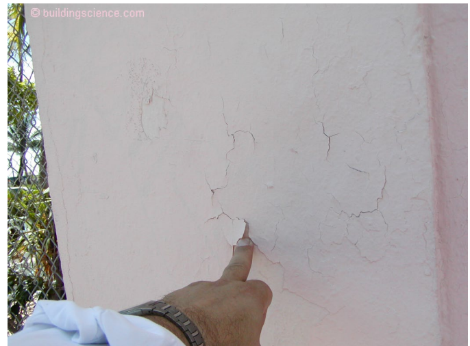
Photograph 6: Impermeable Paint - If the paint on the stucco is too impermeable it bubbles, blisters and peels. The paint on the stucco needs to be greater than 10 perms “wet cup” or it will bubble, blister and peel.
