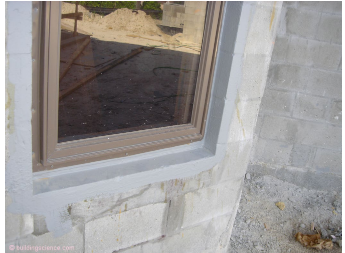
Photograph 9: Fluid Applied Flashing - You absolutely must use a fluid applied coating around the entire perimeter of the rough opening.
