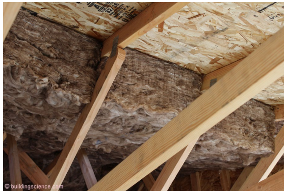
Photograph 9: Fiberglass and Mineral Wool and Cellulose Underside Roof Deck Insulation - Water vapor from the interior passes up through the vapor open insulation and is stored in the wood based roof sheathing – and then driven out by solar radiation. In and then out...in and then out...a “ping” followed by a “pong” leading to an increase in moisture accumulating at the ridge requiring a means of moisture removal.... either air supply and return from the house coupled with a “vapor diffusion port” or a dehumidifier
