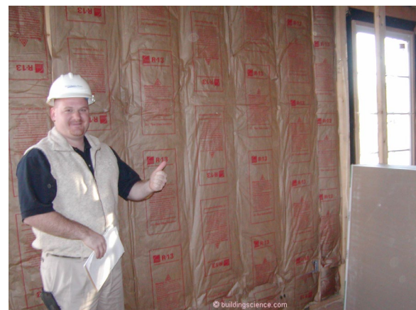
Photograph 11: Faced Insulation Batts – Air flow and convection can be effectively controlled by facers adhered to batt insulation. Note that faced insulation batts should have the facers installed to the “face” of the stud framing – not “inset stapled”. Inset stapling creates voids and air channels that can lead to convective loops and a loss of thermal resistance.
