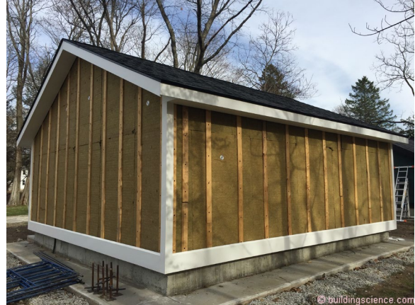
Photograph 3: Mineral Wool Board Insulation – The insulation boards installed on the exterior of framing can act as the thermal control layer...but they need to be coupled with a water control layer, air control layer and vapor control layer...mineral wool board insulation can do only one of the control layers.
