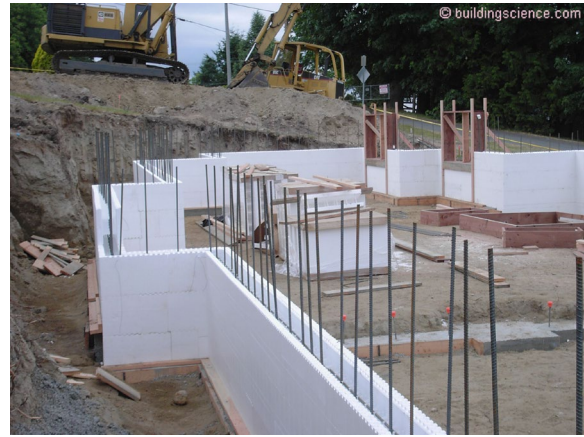
Photograph 5: Insulated Concrete Forms (ICF's) - They can act as the air control layer, vapor control layer and thermal control layer. They need to have a water control layer installed on their exterior or a cladding such as polymer based (PB) stucco directly attached to their exterior face creating a barrier wall mass assembly.
