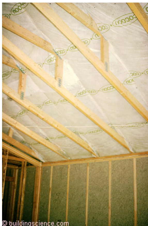
Photograph 12: Netted and Damp Spray Cellulose
