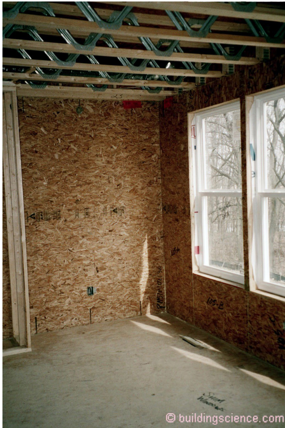
Photograph 4: Structural Insulated Panels (SIP's) - They can act as the air control layer, vapor control layer and thermal control layer but not the water control layer. They need to have a water control layer installed on their exterior.
