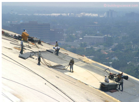
Photograph 7: Spray Polyurethane Foam Roofing - A fluid applied roofing membrane can be applied directly to the ccSPF. The Louisiana Superdome was successfully repaired with this approach after Hurricane Katrina.
