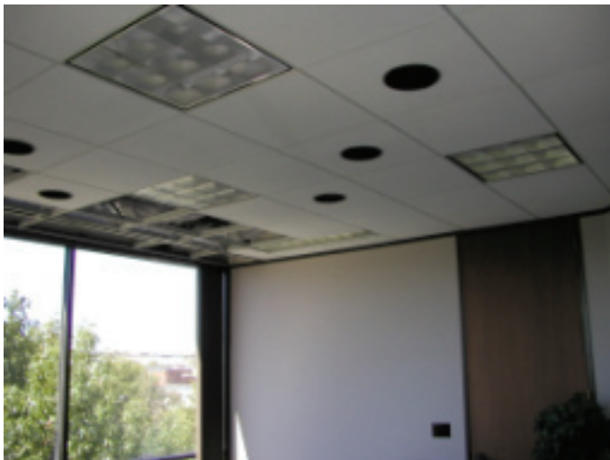
Photograph 1: The Ubiquitous Dropped Ceiling Return Plenum
