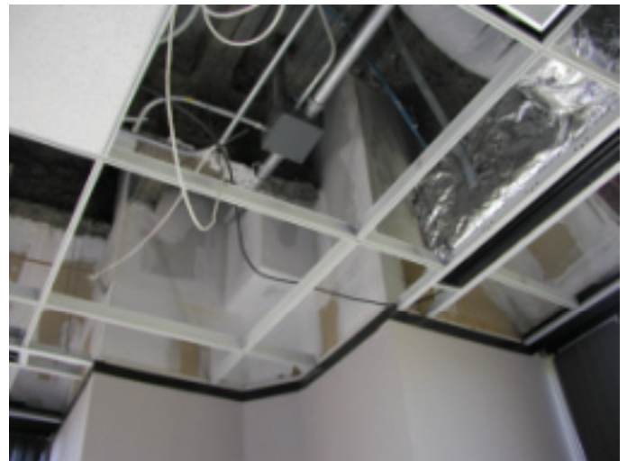
Photograph 3: Retrofit of Closure
