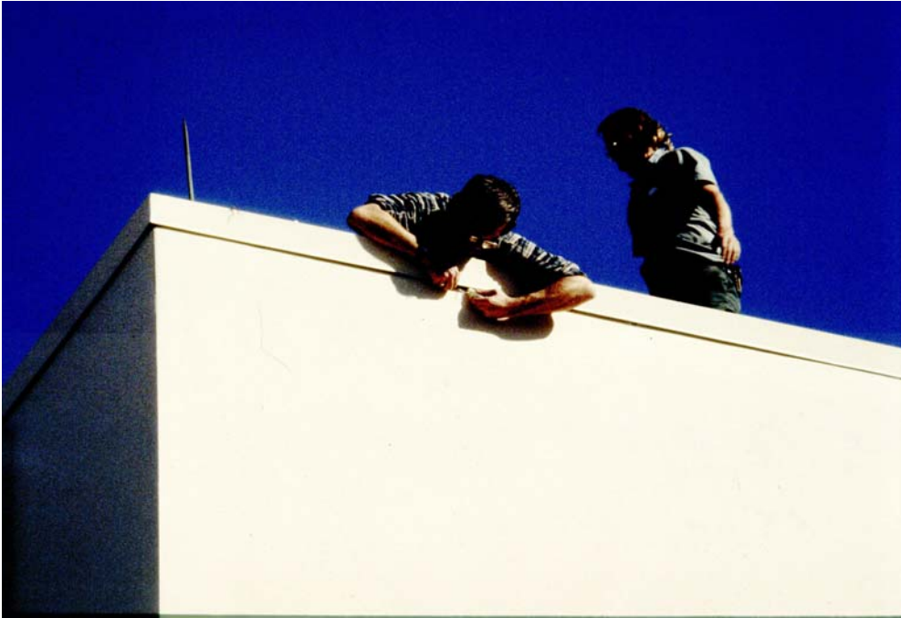
Photograph 4: Parapet Fresh Air Intake
