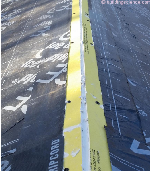
Photograph 1: Vapor Diffusion Port – The vapor diffusion port covering must be non-combustible such as gypsum board.
