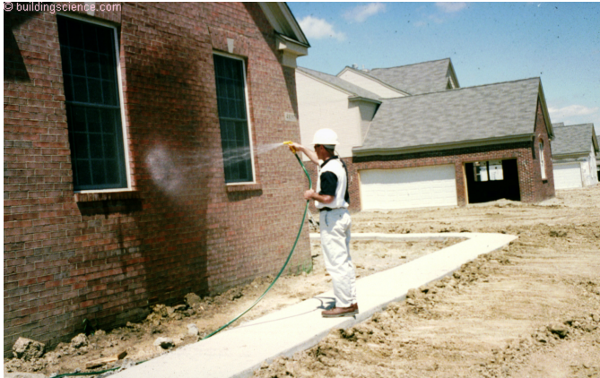
Photograph 1: Water Test - I have tricked a youngster into using an ordinary garden hose to spray water against a brick veneer. This field test follows no approved ASTM protocol.
