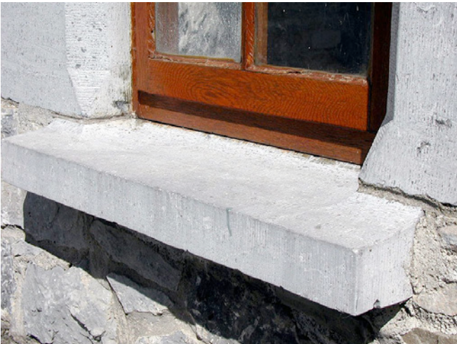
Photograph 5: Old Irish Stuff— Doing it right. Unbelievably beautiful. End dams, a back dam, slopes and a kerf. Wow, wow, wow.
