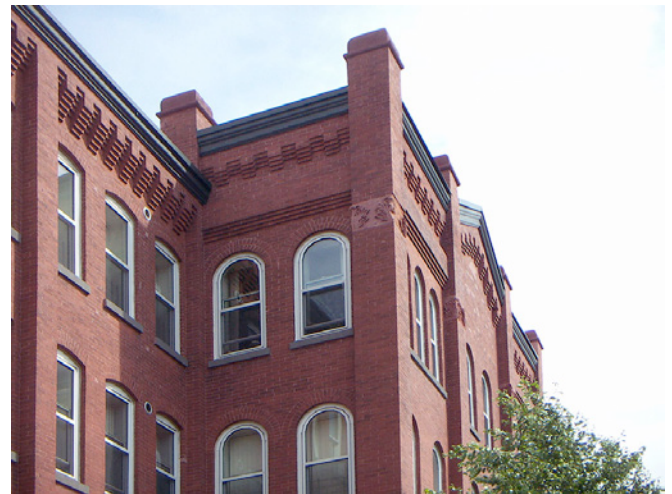
Photograph 8: All Time Favorite —An old brick factory converted to seniors housing with “good brick” on the street side. All the drips, the flashings, the end dams, the back dams, the slopes, the kerfs, the parapet caps were added as unobtrusively as possible. The street side brick—shown here—was cleaned. Notice the fabulous parapet that was added with the drip cap.
