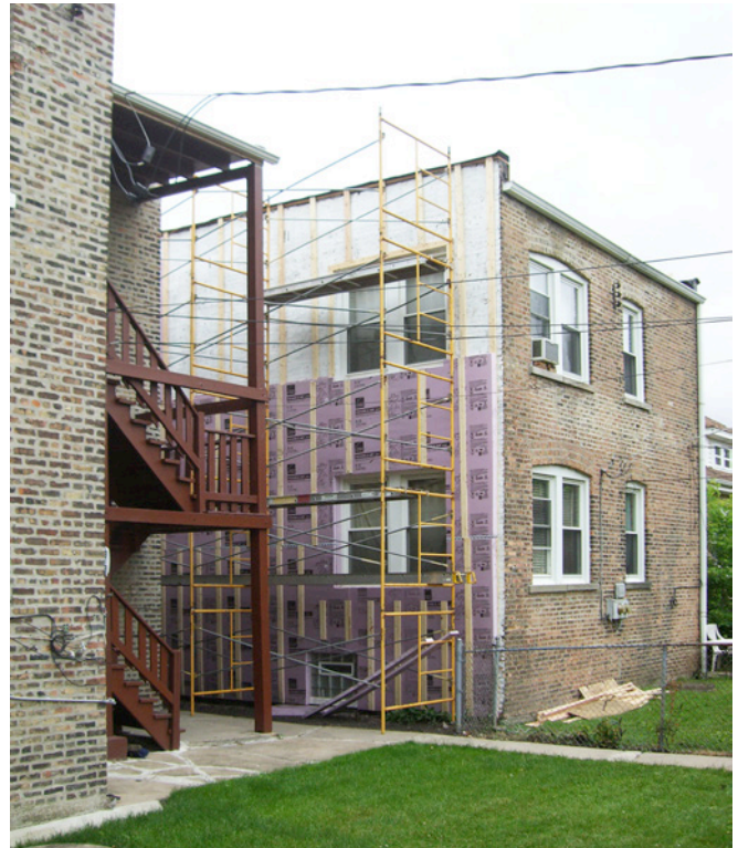
Photograph 13: House-Sized Sequencing —With house-sized buildings you also work you way around the sides.
