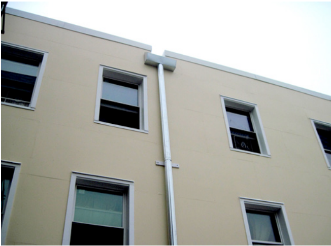
Photograph 11: Scupper Detail —You have to drain the roof.
