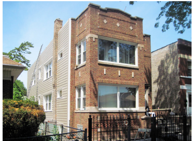
Photograph 14: Finished House Overclad —In many cases the exterior insulation only wraps three sides of the four sided “box”. The “street side” is left undone for “aesthetic” reasons.
