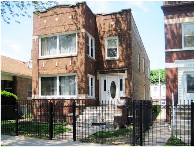
Photograph 2: House-Sized—Uninsulated masonry building
