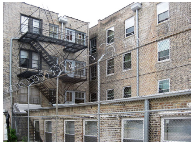
Photograph 1: Jumbo-Sized —Uninsulated masonry building
