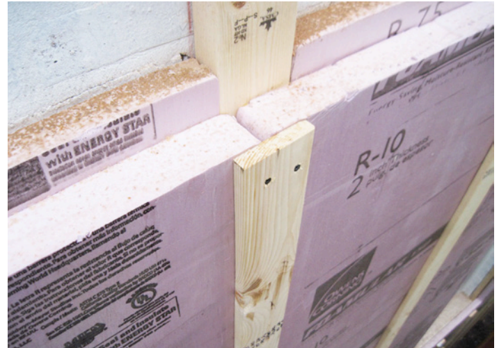
Photograph 3: "Secret" Trick - 2x4 wood furring "on the flat"— once you attach that, everything else attaches to that, and it is easy sailing. And it is not a big deal to attach wood furring directly to masonry or to concrete—we know how to do that.
