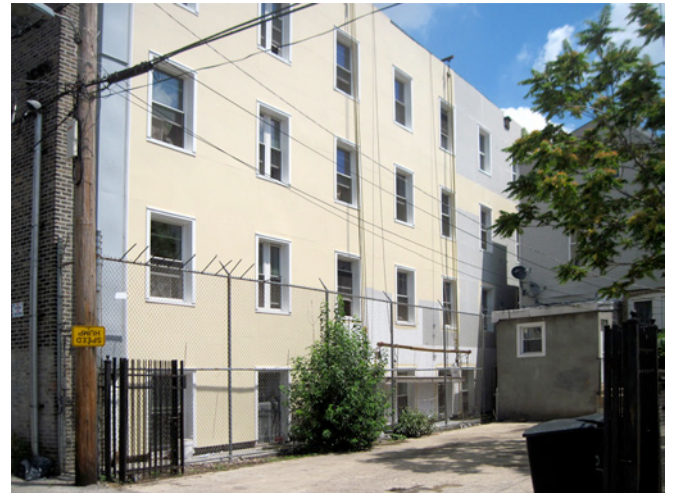
Photograph 9: Fiber cement Panels —Fireproof and pretty robust.
