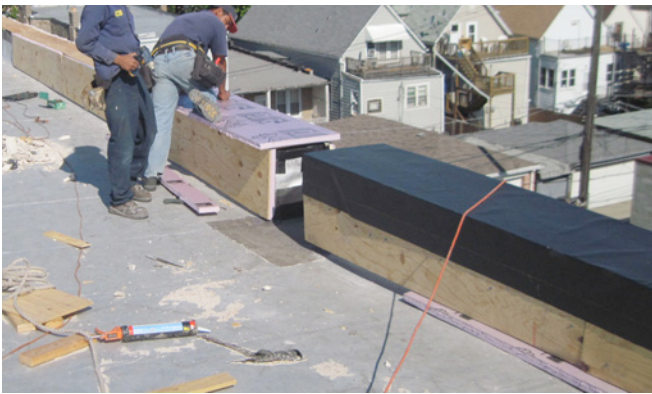
Photograph 5: Parapet Insulation —Don’t forget to slope the parapet to the interior.
