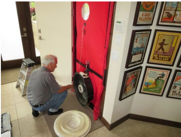
Figure 44: Building depressurization while spraying
