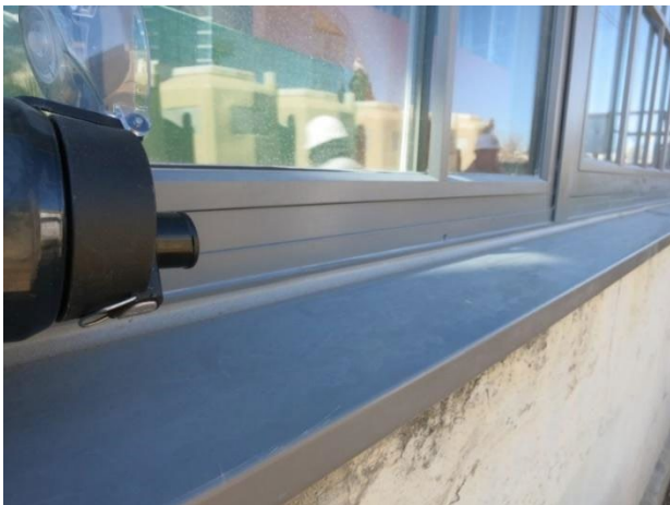
Figure 13: Water testing a sill with acceptable slope
