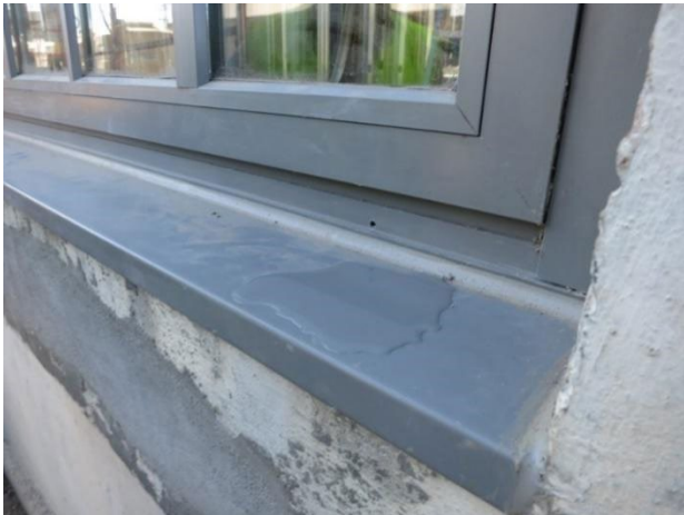
Figure 12: Water testing a sill with minimal slope
