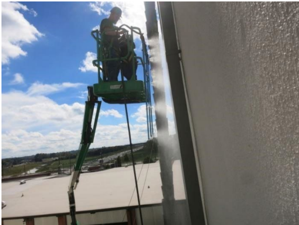
Figure 36: Window test spray rack in operation
