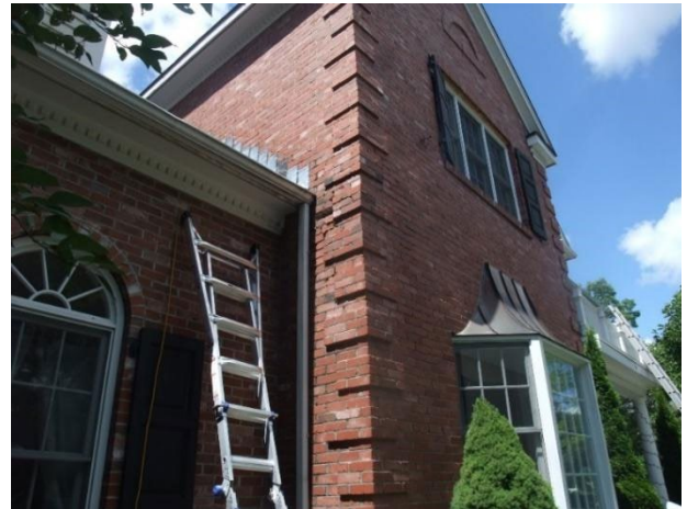
Figure 2: Roof-to-wall interface at brick building
