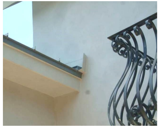
Figure 6: Kickout flashing in stucco building
