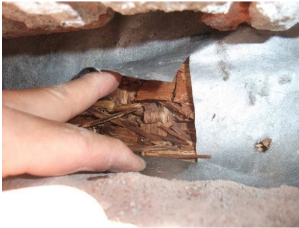
Figure 4: OSB behind housewrap
