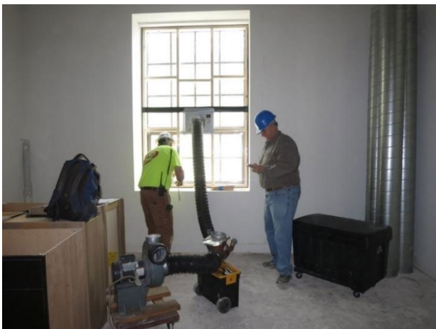
Figure 37: Window interior depressurization rig
