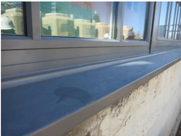
Figure 14: Water testing a sill with acceptable slope
