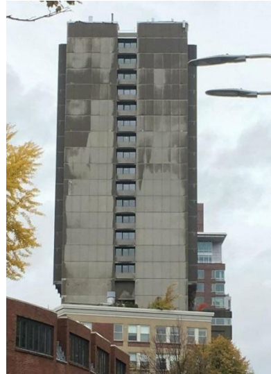
Figure 10: Water deposition patterns on tall buildings
