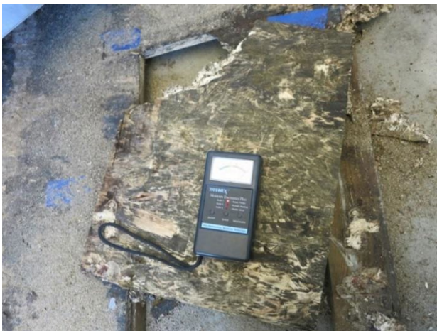
Figure 31: Tramex measurement of subfloor
