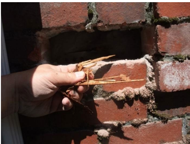
Figure 5: OSB strands hand-removable
