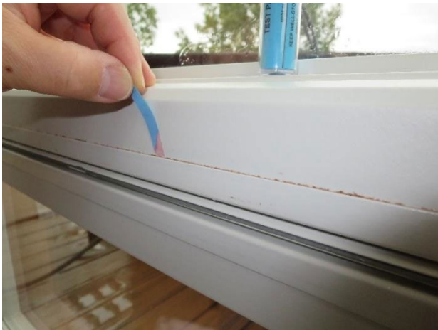
Figure 48: Water indicator paper to probe joint
