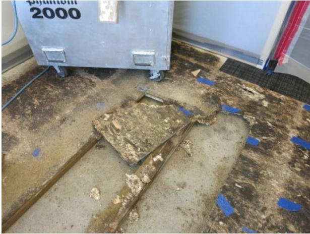
Figure 30: Disassembly of floor over slab
