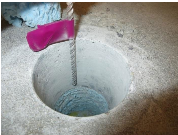
Figure 33: Drilled hole to lower part of slab
