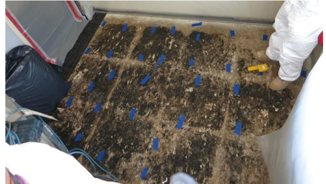
Figure 28: Discoloration matches carpet tile patterns
