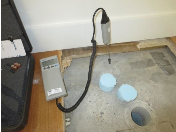
Figure 32: Slab internal T/RH measurement
