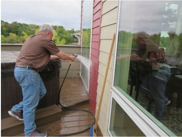
Figure 43: Water spray testing windows
