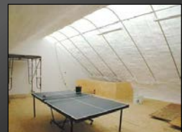
After the interior finish coating
