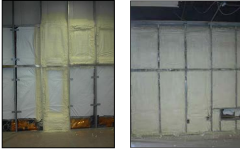
The drainage plane was sealed with SPF during the insulation installation
