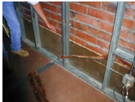
Copper through-wall flashing was found at the base of the wall
