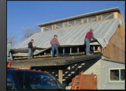
Fabric installed - before stretching
