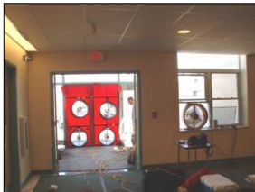
Compliance Test – No masking of Mechanicals
