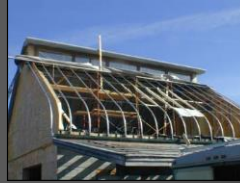
Preparing to install the roofing membrane on the lower-side bows
