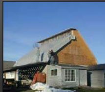
Wrapping the fabric at the gable end prior to stretching
