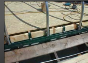
Unistrut frame at the top of the bows
