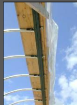
Unistrut frame at the top of the bows
