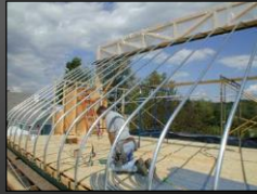
Lower side bows in place
