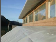
Installing the membrane below the monitor windows
