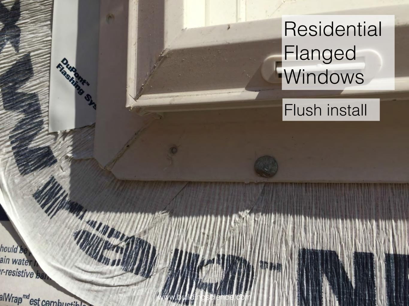
Fold and tape WRB over self adhered membrane flashing at head
