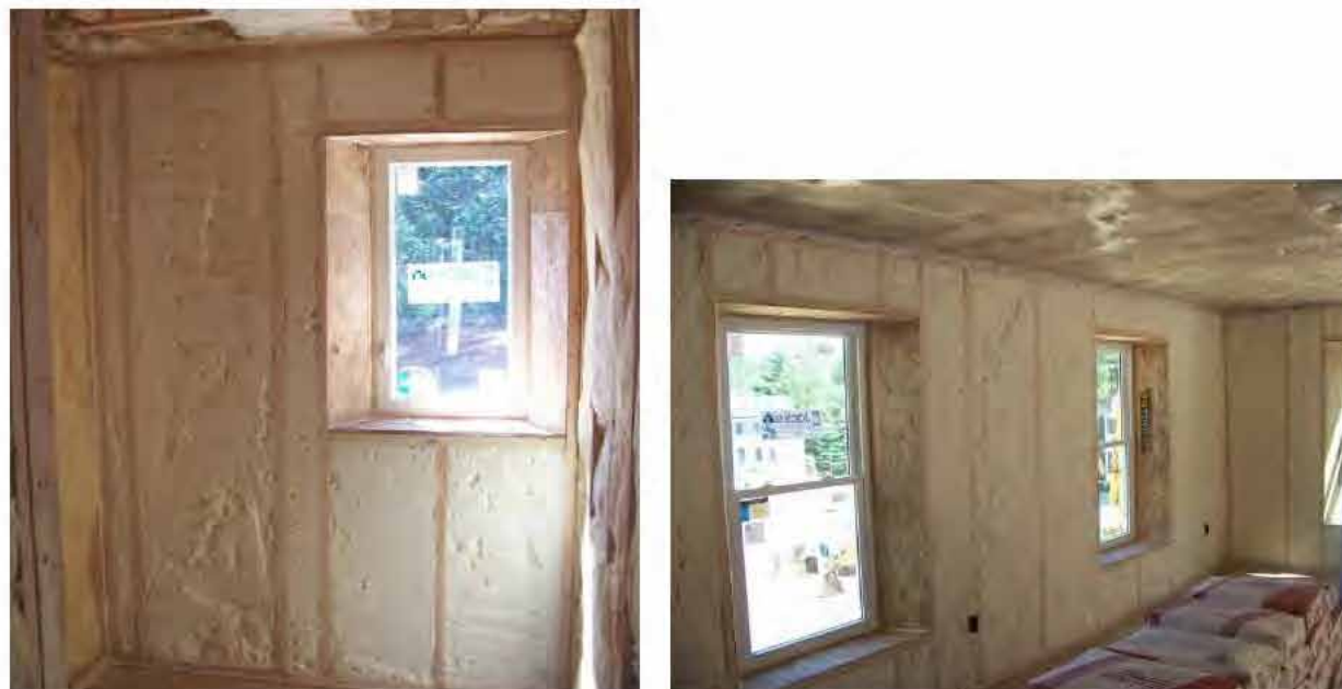
Figure 44. Typical installation of ½ lb/ft 3 spray foam in double-stud walls
