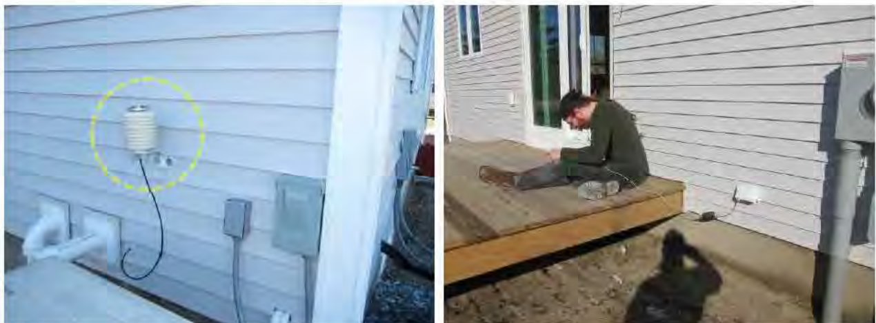
Figure 53. (L) Exterior T/RH sensor; (R) data collection from exterior connection port
