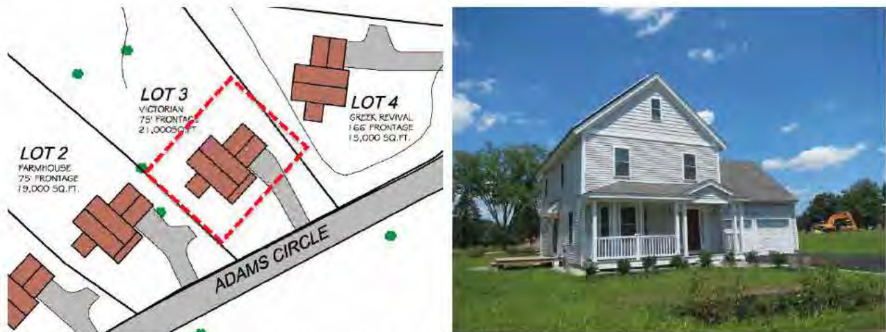
Figure 45. Overhead (L) and front (R) views of Lot 3 test house
