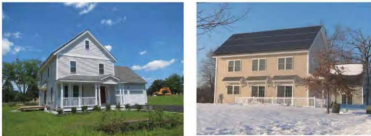
Figure 21. (L) Exterior of houses at Devens; (R) Easthampton
