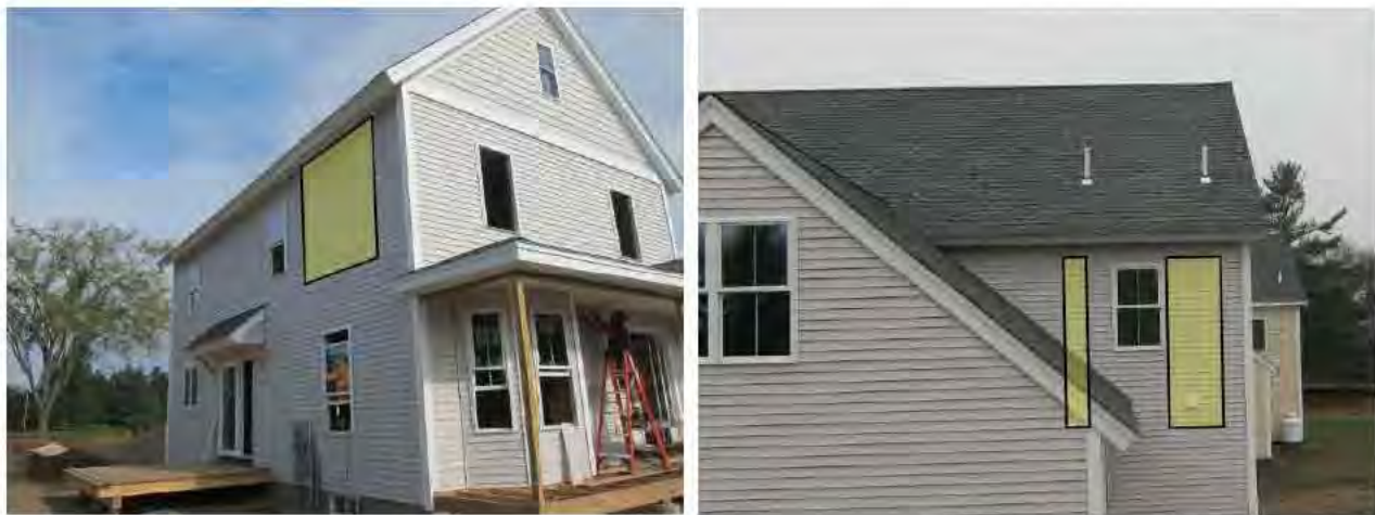
Figure 47. Test wall locations shown on exterior of house; south (L) and north (R) orientations
