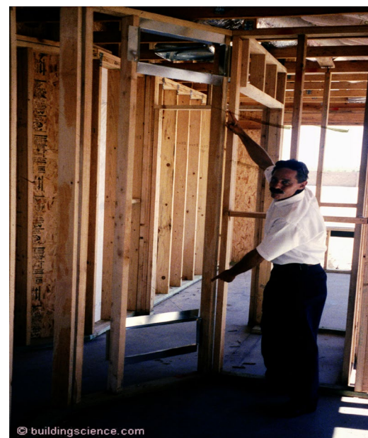
Photograph 4: Transfer Grilles - Grille high on one side, low on the opposite side to control light and noise transfer.
