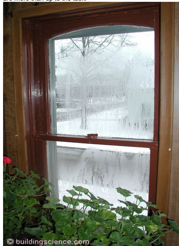
© buildingscience.com Photograph 12: Fabulous Windows - With “fabulous” windows we can get rid of the supply return ducts all together. Having said that, we will still need some means of distributing ventilation air. Fully ducted HRV’s and ERV’s are more than up to the task.
