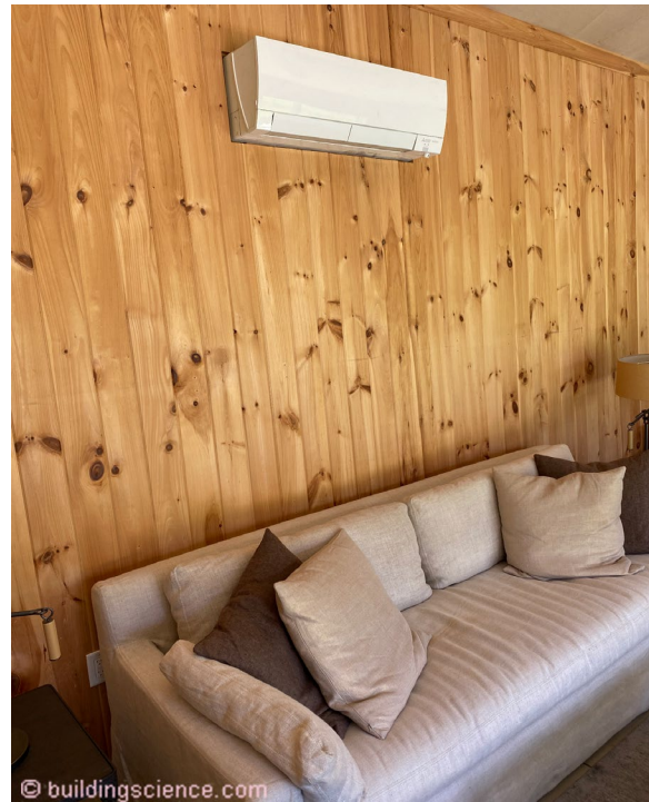
© buildingscience.com Photograph 11: Fabulous Windows - With “fabulous” windows we can get rid of the supply return ducts all together. Having said that, we will still need some means of distributing ventilation air. Fully ducted HRV’s and ERV’s are more than up to the task.
