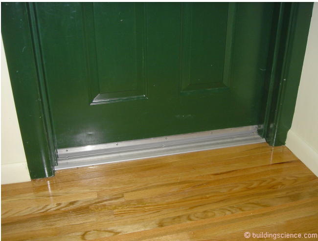
© buildingscience.com Photograph 6: Weather-Stripped Door – a beautiful thing if you are worried about fires.
