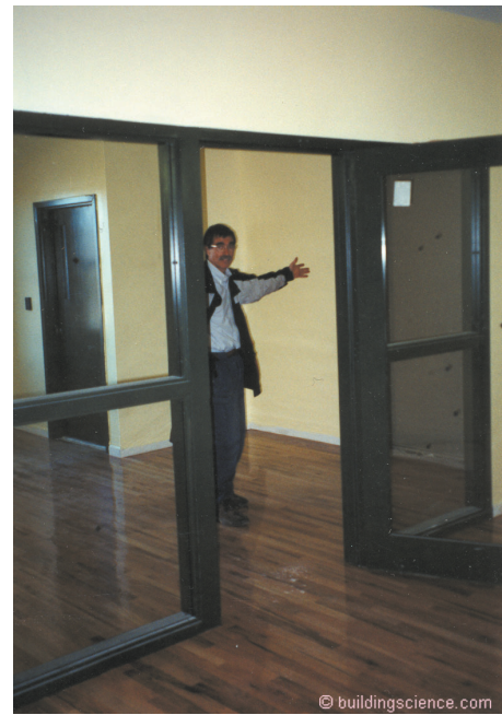
© buildingscience.com Photograph 8: Elevator Lobby – enclosed in a vestibule, or “air lock” that isolates the vertical communication from the horizontal communication.
