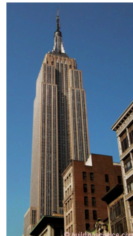
Photograph 2: Old School – magnificent depression era building with operable windows. Not bad for a bunch of geezers, eh?
