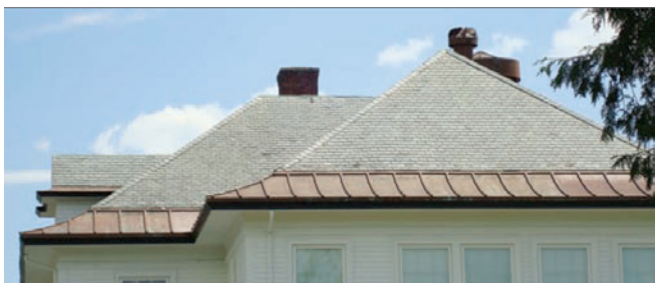
Photograph 2: New England Slip Surface —Older buildings in New England use metal “slip” surfaces to get the snow to slide off the roof, preventing the ice dam from occurring at the roof edge.
