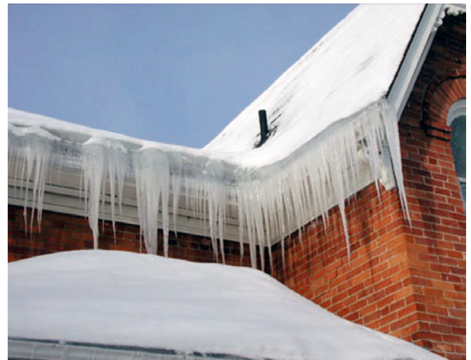
Photograph 1: Ice Dam —Beautiful, but bad, and sometimes dangerous. Folks die every year when big ones fall on them, or when they fall off roofs trying to get rid of them.
