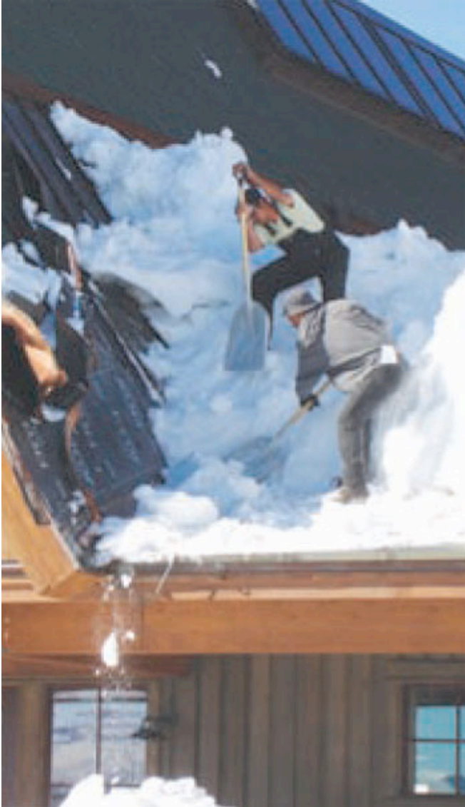
Photograph 10: Australians to the Rescue —They play football without pads. They are fearless, and they make lifelong friends. They also damage your roof when you get them to hack away the ice dams.
