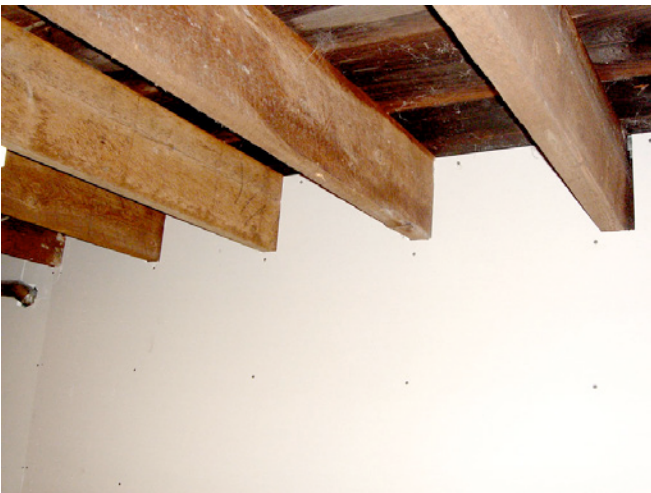
Photograph 17: Gypsum Board Protection Layer —Gypsum is made from a type of rock—and rocks don't burn—this is a good thing.
