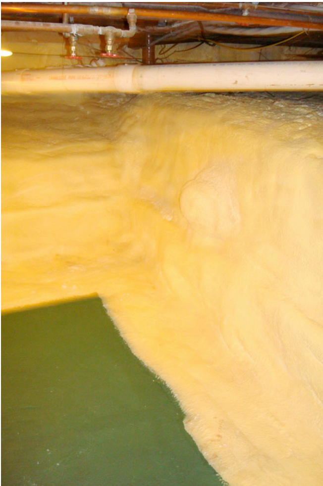
Photograph 7: All Done —The slab was painted to make it look pretty. Remember “green” means environmental.
