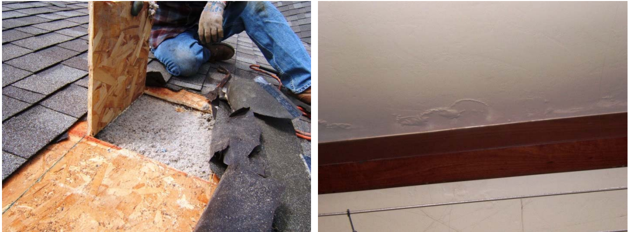
Figure 12. Dry sheathing lower at roof (left); interior ridge conditions (right)
