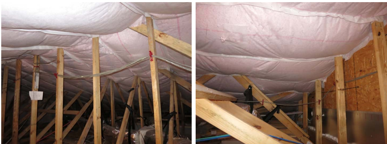
Figure 18. Typical completed attic conditions at ridge (left) and roof-to-wall (right)
