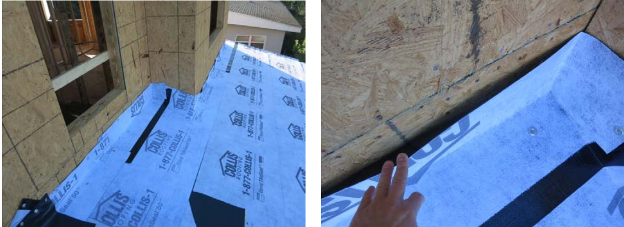
Figure 46. Construction image of roof-wall interface self-adhered membrane (Location E)
