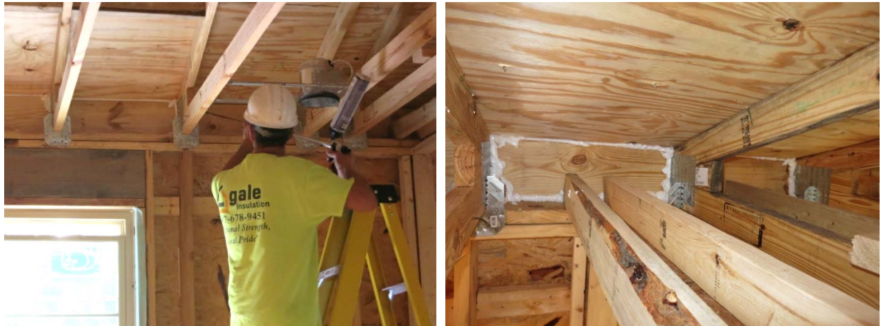
Figure 19. Air sealing roof-to-wall connection; note 2x blocking and single-component foam
