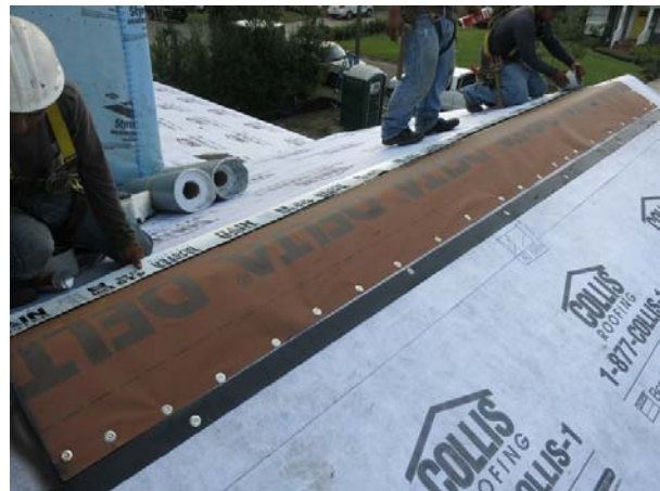
Figure 24. Open slots for vapor diffusion vent (left), diffusion vent membrane (right)
