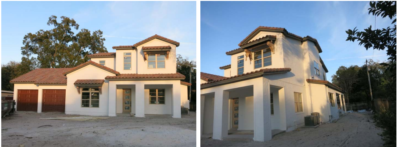
Figure 14. Front and side views of Orlando-area test house
