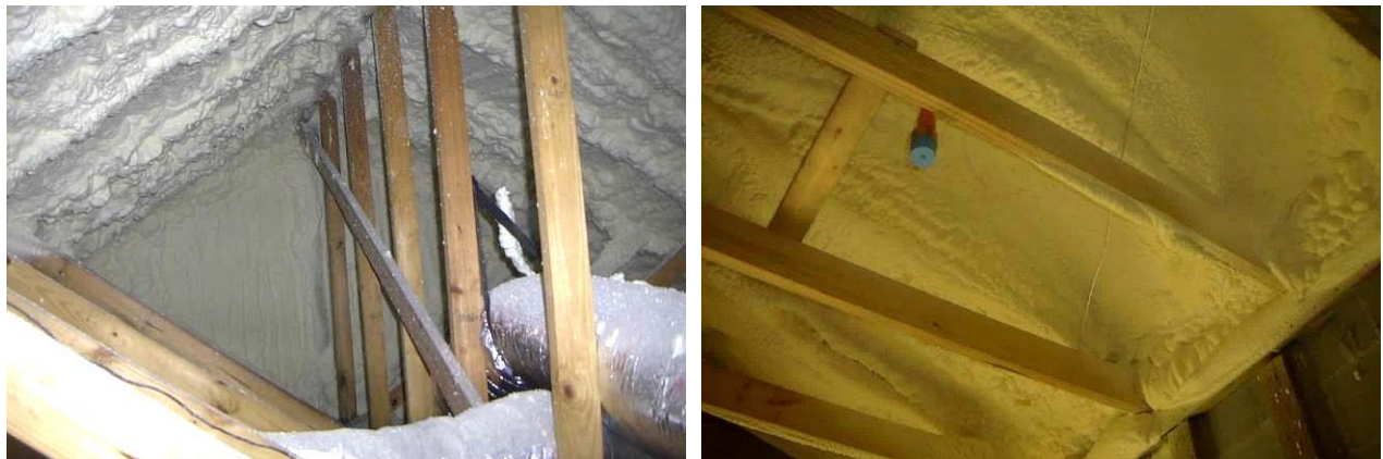
Figure 1. SPF unvented roofs
