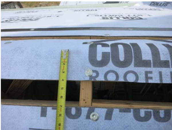
Figure 24. Open slots for vapor diffusion vent (left), diffusion vent membrane (right)
