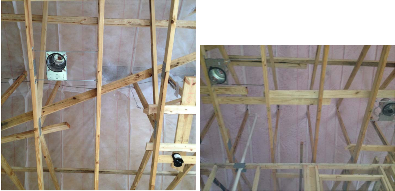
Figure 17. Boxed netting insulation system before (left) and after (right) insulation blowing
