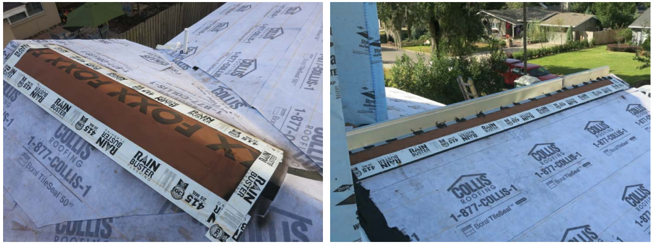
Figure 25. Completed diffusion vent (left); installation of ridge metal (right)
