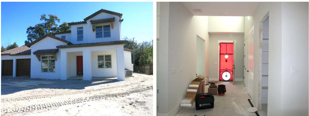
Figure 34. Air leakage (single blower door) testing of the tile roof test house
