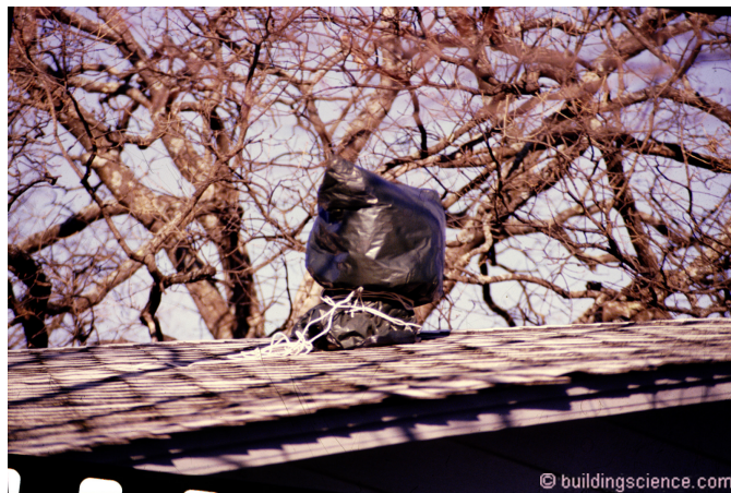
Photograph 5: Civilian Solution – Plastic garbage bag handles the turbine vent problem.
