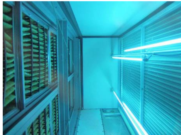
In-Duct/Coil UVGI
