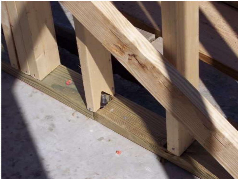
Anchor Bolt Placement
