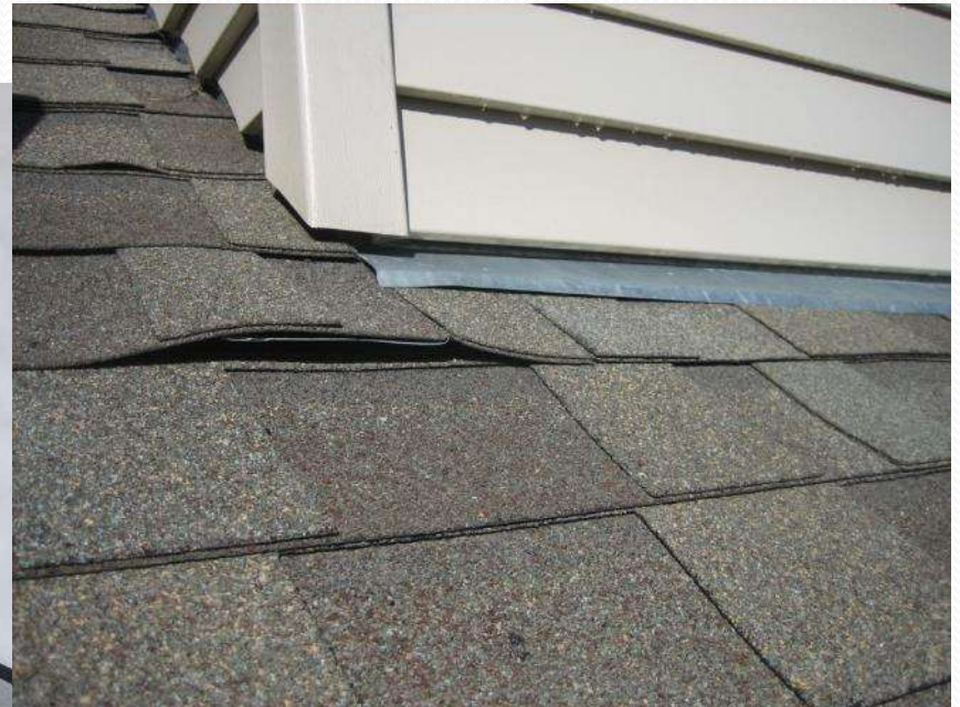
Roof-wall flashing
