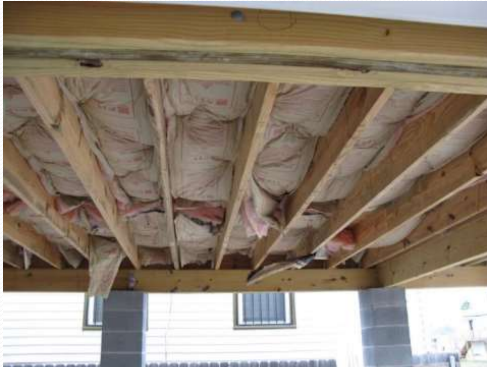
subfloor fiberglass insulation
