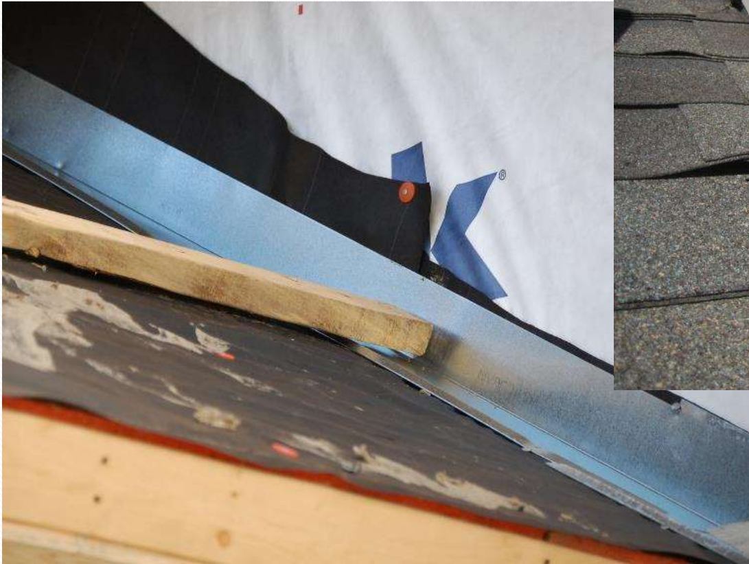
Roof-wall flashing
