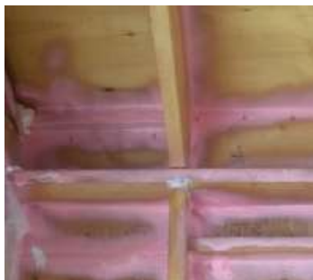
Sealers w/ backup structure
